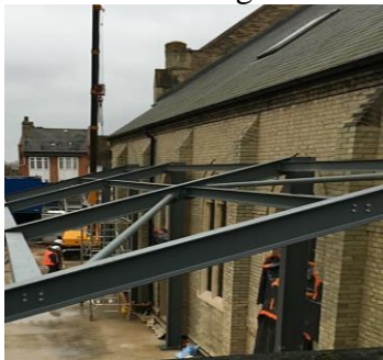
The frame erection is started
