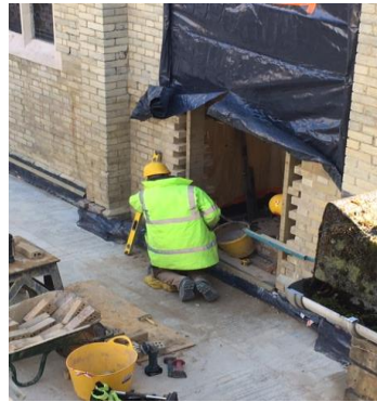
Andy matches the bricks for the entrances into the church
