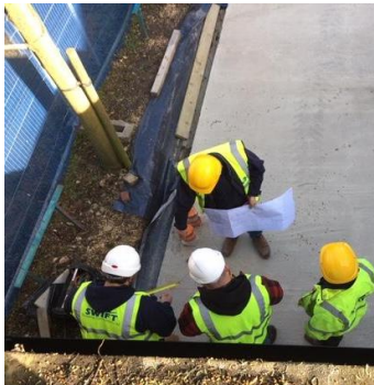
David confirms the position for the first steel girder
